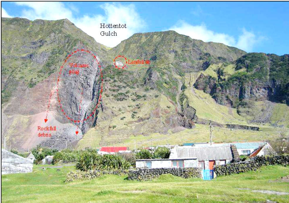
Figure 9 - The Main Cliffs behind the settlement with the areas most vulnerable to rockfalls annotated, most notably the volcanic plug previously identified by Dunkley (2002) as a potential hazard. The recent landslide scar (August 2004) at around 400m in Hottentot Gulch is also marked. (Photograph by the author)
